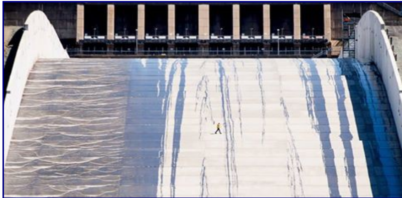
Oroville Dam Spillway
