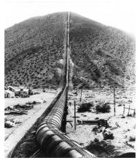
One of the most significant features of the aqueduct is known as the Jawbone Siphon. It's an example of the riveted steel pipelines that cross deep and wide canyons along the aqueduct route. Considered one of the most challenging projects, the pressure siphon piping is made up of different diameters to help move water across vast stretches of the canyon.
