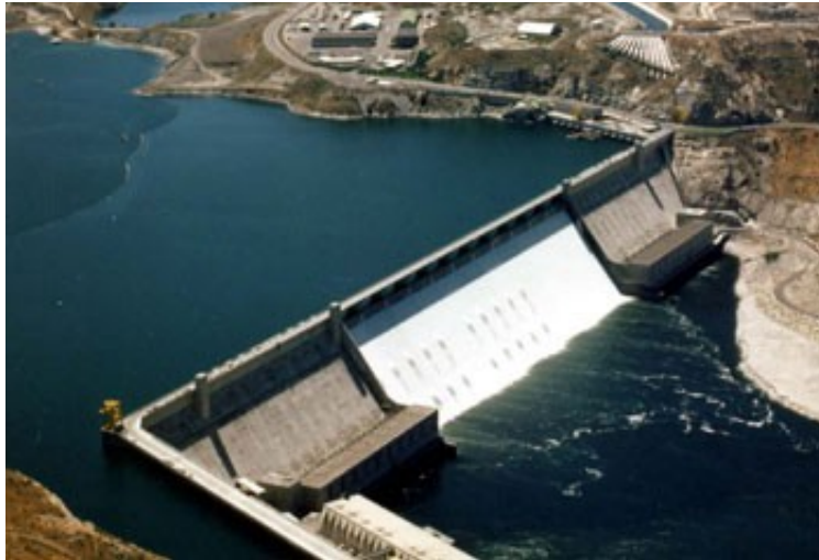
Grand Coulee Dam, on the Columbia River west of Spokane, Washington, is one of the largest structures ever built by mankind--a mass of concrete standing 550 feet high and 5,223 feet long--or just shy of a mile. Bureau of Reclamation
