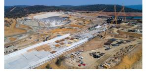
A drone provides an overview of the recovery effort on the upper chute of the Lake Oroville main spillway and the emergency spillway splashpad on the hillside above the secant pile wall at the Butte County, California site. DWR/2018
