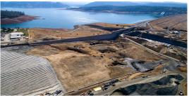
A drone provides a bird's-eye view of the Lake Oroville emergency spillway and the recently added roller compacted concrete (RCC) splashpad as crews start the second phase of construction on the RCC splashpad on the hillside above the secant pile wall at the Butte County, California site.
