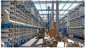
Workers paint the scaffolding for the roof that will cover the walls of filters used in desalination and are in place at Poseidon Water's desalination plant site in Carlsbad. (File photo)
