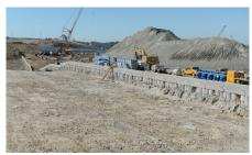
The cut-off wall below the emergency spillway weir for Oroville Dam is designed to stop uphill erosion like that which prompted evacuations in February 2017. (Bill Husa – Mercury-Register)
