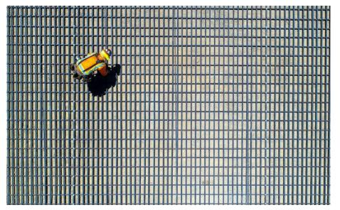
A worker assembles structural rebar panels for concrete that will be placed on the Lake Oroville main spillway during Phase 2 of the recovery efforts at the Butte County, California site. DWR/2018
