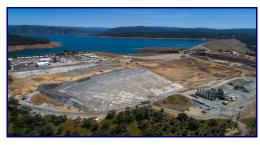
An aerial view of the Lake Oroville spillways construction site that shows progress of the roller-compacted concrete (RCC) splashpad that will armor the hillside between the emergency spillway and the secant pile wall in Butte County, California. Photo taken May 7, 2018.
