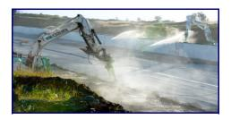
Excavators from Ferma Corporation begin removing the temporary roller-compacted concrete (RCC) sidewalls of the Lake Oroville main spillway in Butte County, California. These temporary walls will be replaced with structural concrete walls later this year. Photo taken May 8, 2018. Kelly M. Grow/ California Department of Water Resources, FOR EDITORIAL USE ONLY
