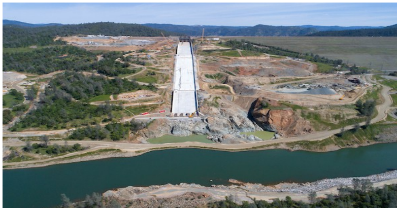
Drone view of the main spillway at Lake Oroville, March 29, 2018 (DWR)
