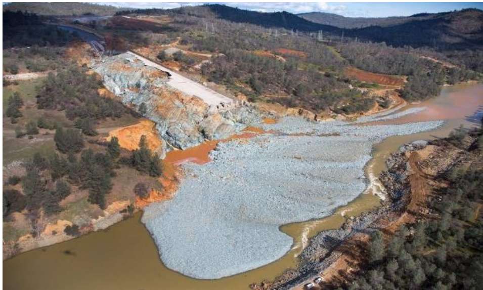
The debris from the damaged spillway fill the Feather River
