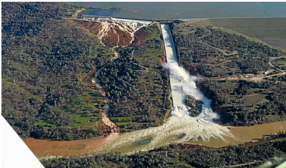
Aerial photo taken Sunday morning, February 12, shows water running over the emergency spillway,
