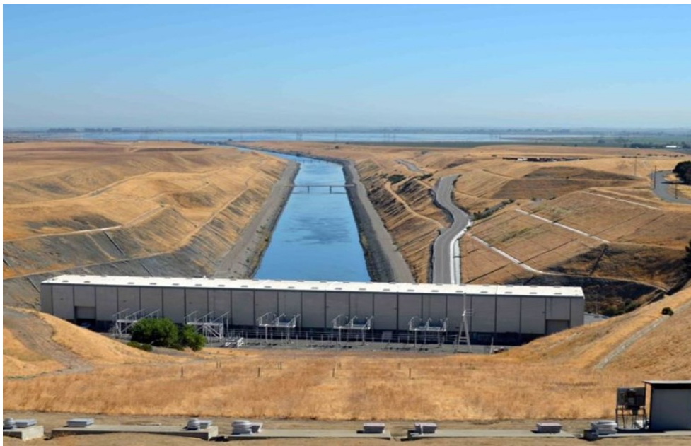
Harvey O Banks Pumping Plant near Tracy, part of the State Water Project. Photo / Curtis Jerome Haynes
