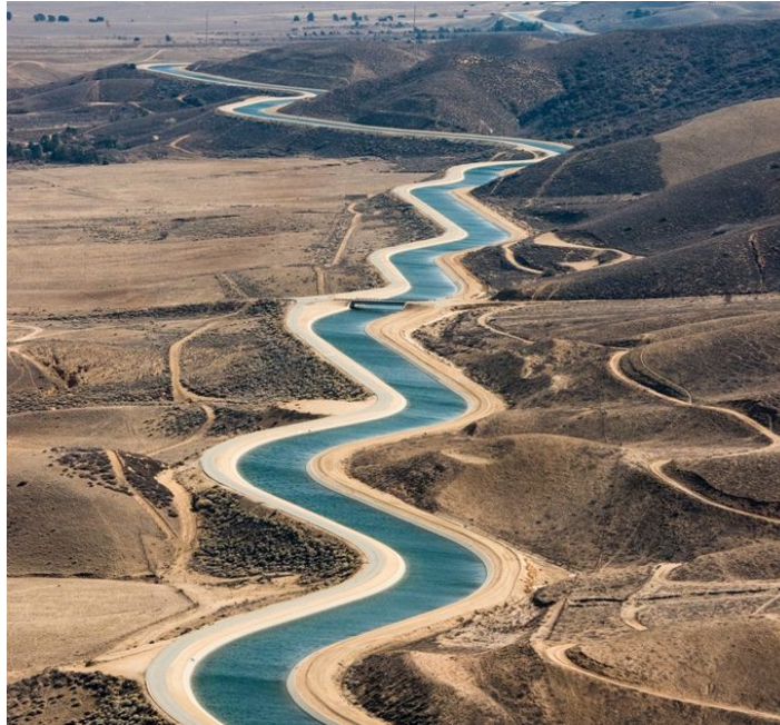
The California Aqueduct. (Photo: CA State Water Project)
