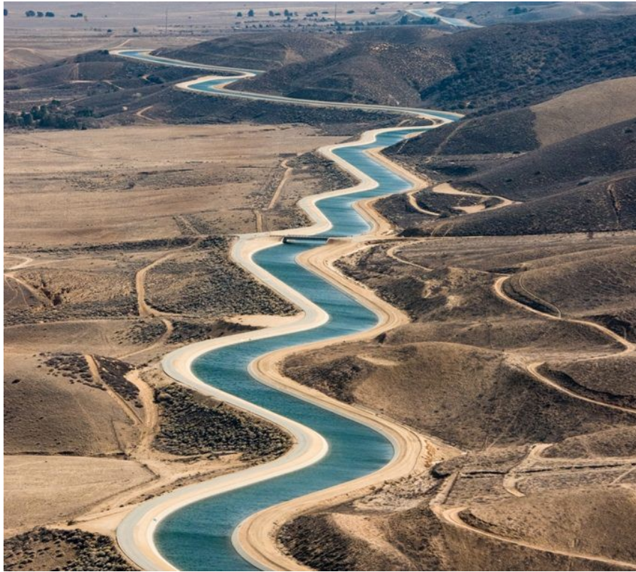
The California Aqueduct. (Photo: CA State Water Project)
