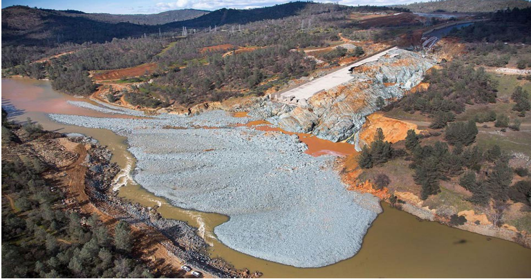
Figure 1. Debris fills the Feather River from the damaged spillway of California's Oroville Dam, the nation's tallest dam, after its near-collapse in February 2017. The Oroville incident forced the evacuation of nearly 190,000 people and cost $1.1 billion in repairs. (Image credit: California Department of Water Resources )
