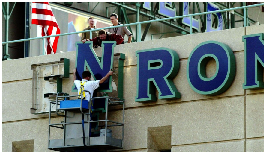
Enron being dismantled
